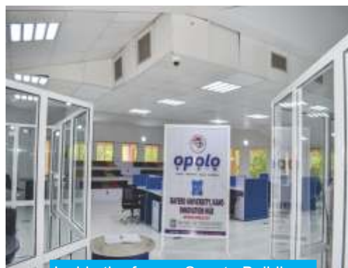
Inside the former Senate Building
